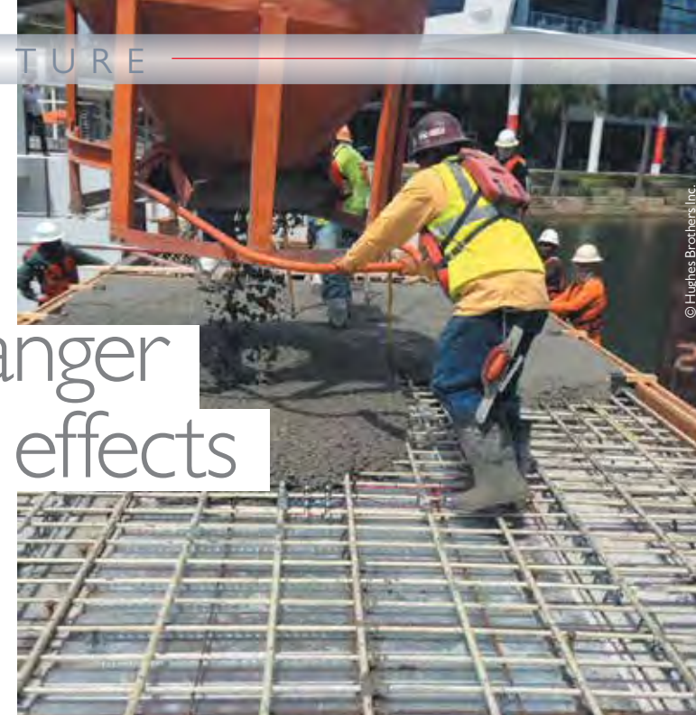
Pedestrian bridge, University of Miami campus August 2015, © Hughes Brothers Inc.
